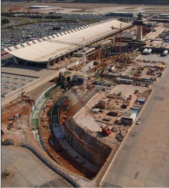
Cut and Cover Tunnel and Main Terminal Station
